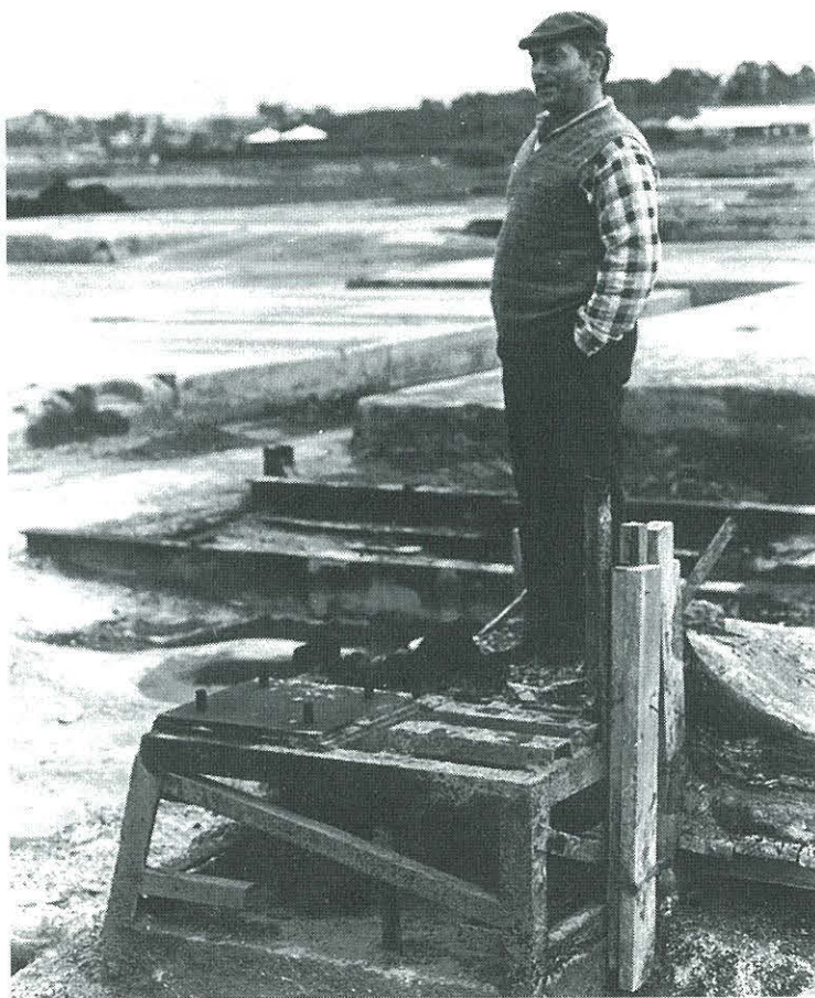
The late Joe Tripodi, concrete pipe worker, reflects on the ruins of his old workplace, now part of the History of the Land Trail at Melbourne's Living Museum of the West. 1987.
